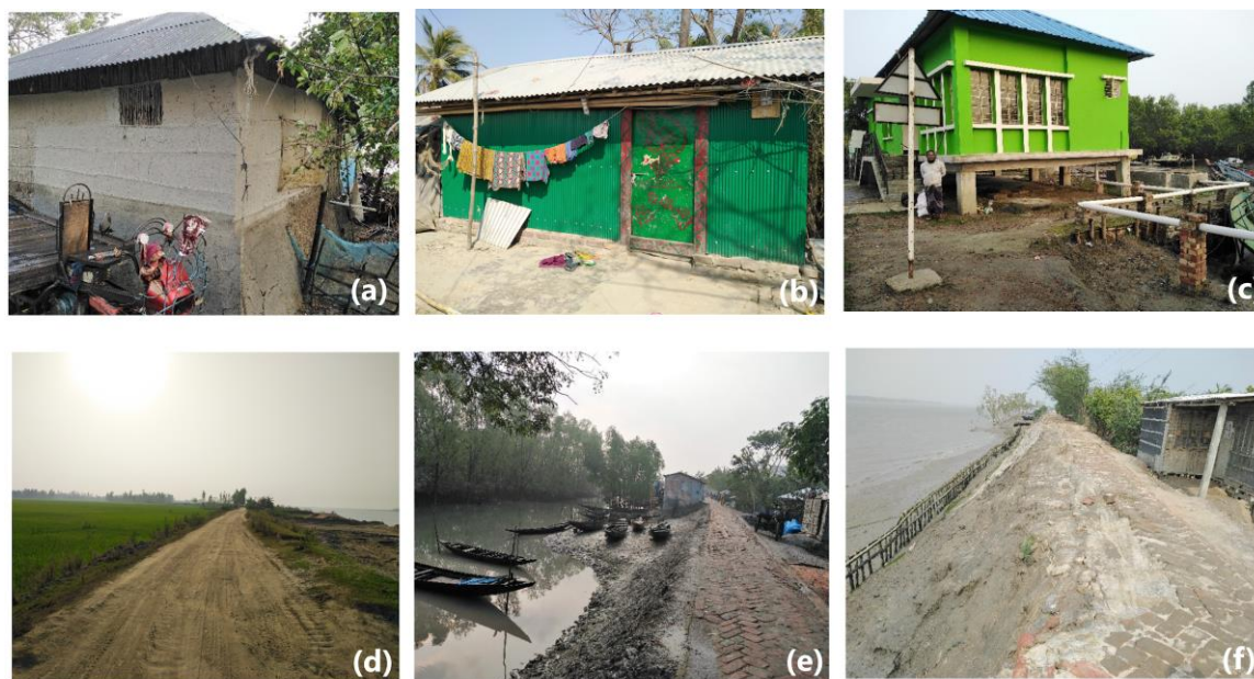
Typical building and road categories in the study area - (a) Kutchha house (b) Semi Pucca house (c) Pucca house (d) Mud road (e) Single brick road (f) Double brick road.
